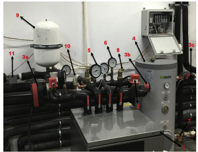
Fig. 2. The components of heat pump.
