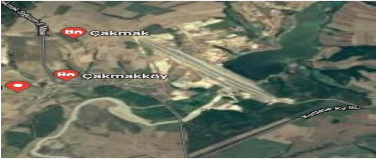
Şekil 5.11.Çakmak Barajı, Kaynak: ( https://www.google.com.tr/maps/search/%C3%A7akmakbaraj%C4%B1/@41.3791293,26.658975,6421m/data=!3m1!1e3,22.04.2019 )
