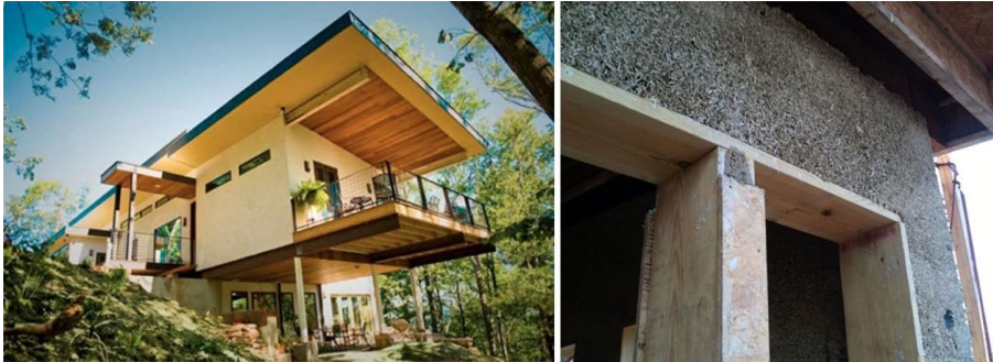
Figure 14. A Hempcrete residential building constructed in Asheville, North Carolina, by Hemptech Global (Hemptechglobal, 2019).
