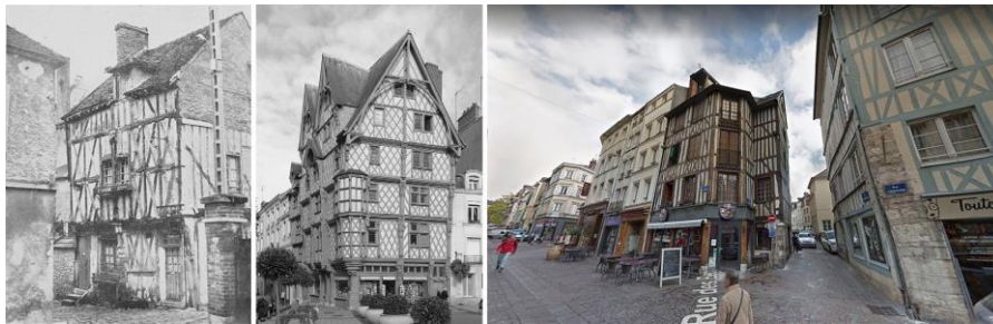
Figure 10. a) The first Hempcrete use in the renovation of Nogent-sur-Seine, France; b) Maison d'Adam, Angers, France, renovated in 1994 (Chevreuil, 1966); (Google Map, 2019); (Gołębiewski, 2017).
